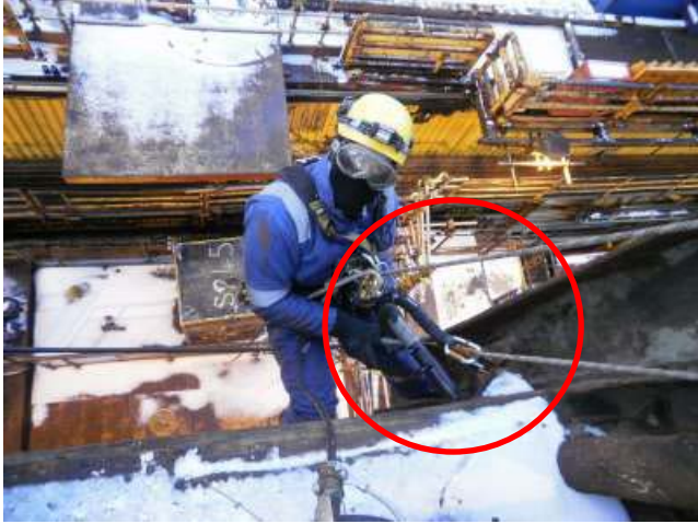
Cold weather needle gunning on the Brent Delta using an 'ID' descender and 'ASAP' back-up device.....
