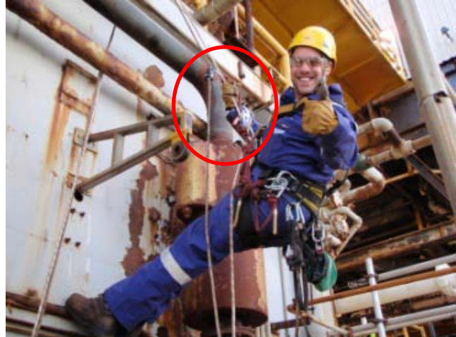
....and using a 'Stop' descender and 'Shunt' as a back-up device in sunnier climes on the Brent Bravo!
